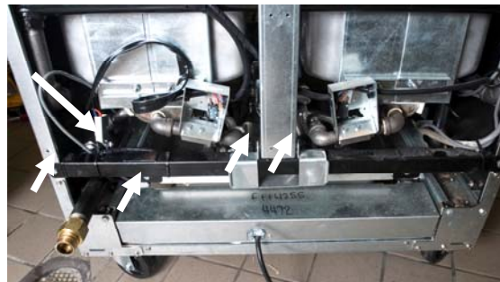
Figure 1: The square oil-return manifold is visible. The port on the left side (marked by down arrow) is removed and the bolts (marked by arrows) supporting the manifold are removed or loosened. The right side manifold bolts are loosened.
