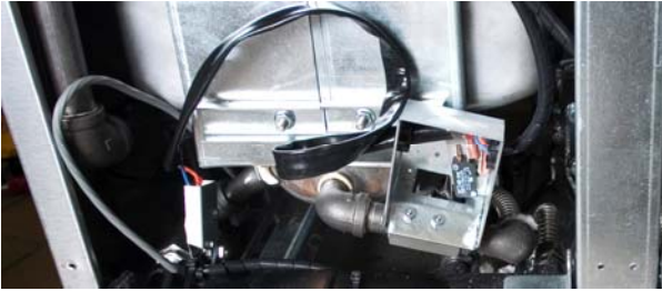
Figure 4 The rear valve switch is shown in place. It is wired in parallel with the existing switch, using piggyback terminals.
